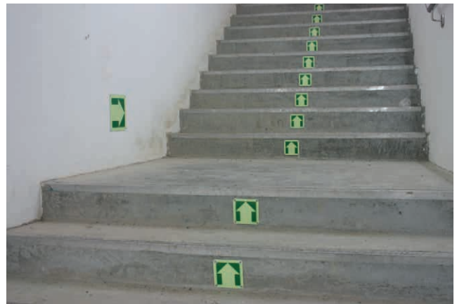
Marine Coastal Expressway - Singapore
